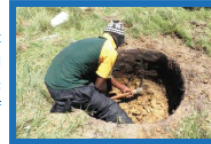
Franchisees at work - digging holes for new toilets.
